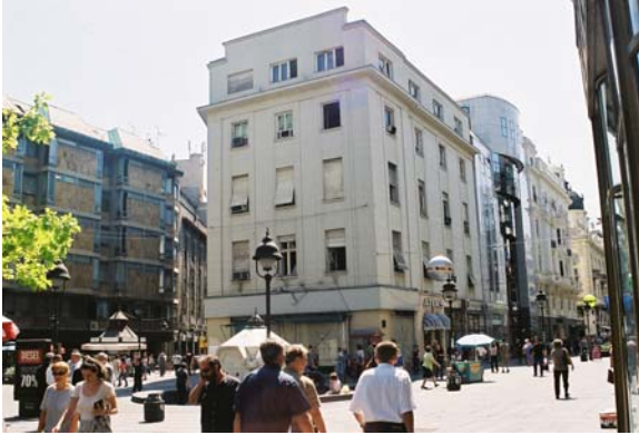
The former USIS Library occupied a prominent location in the city center of Belgrade, Serbia.
