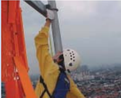
An IBB antenna maintenance technician, known as a "rigger," works on an IBB antenna tower in Indonesia.
